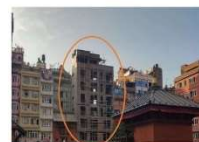
Fig: Newly constructed building without separation gap
